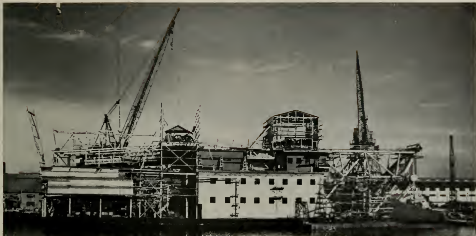
Tin mining dredge Stuyvesant being completed at outfitting pier Tampa Shipbuilding Company, Inc., Tampa, Florida.
